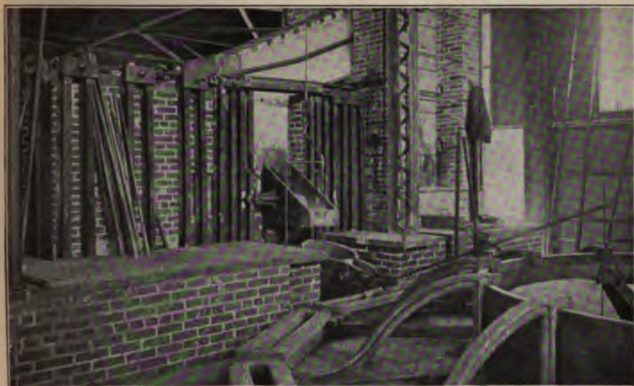
WALKER'S IMPROVED CASTING APPARATUS. Showing Receiving Ladle, Deflector, Molds, and Turntable Arms,
